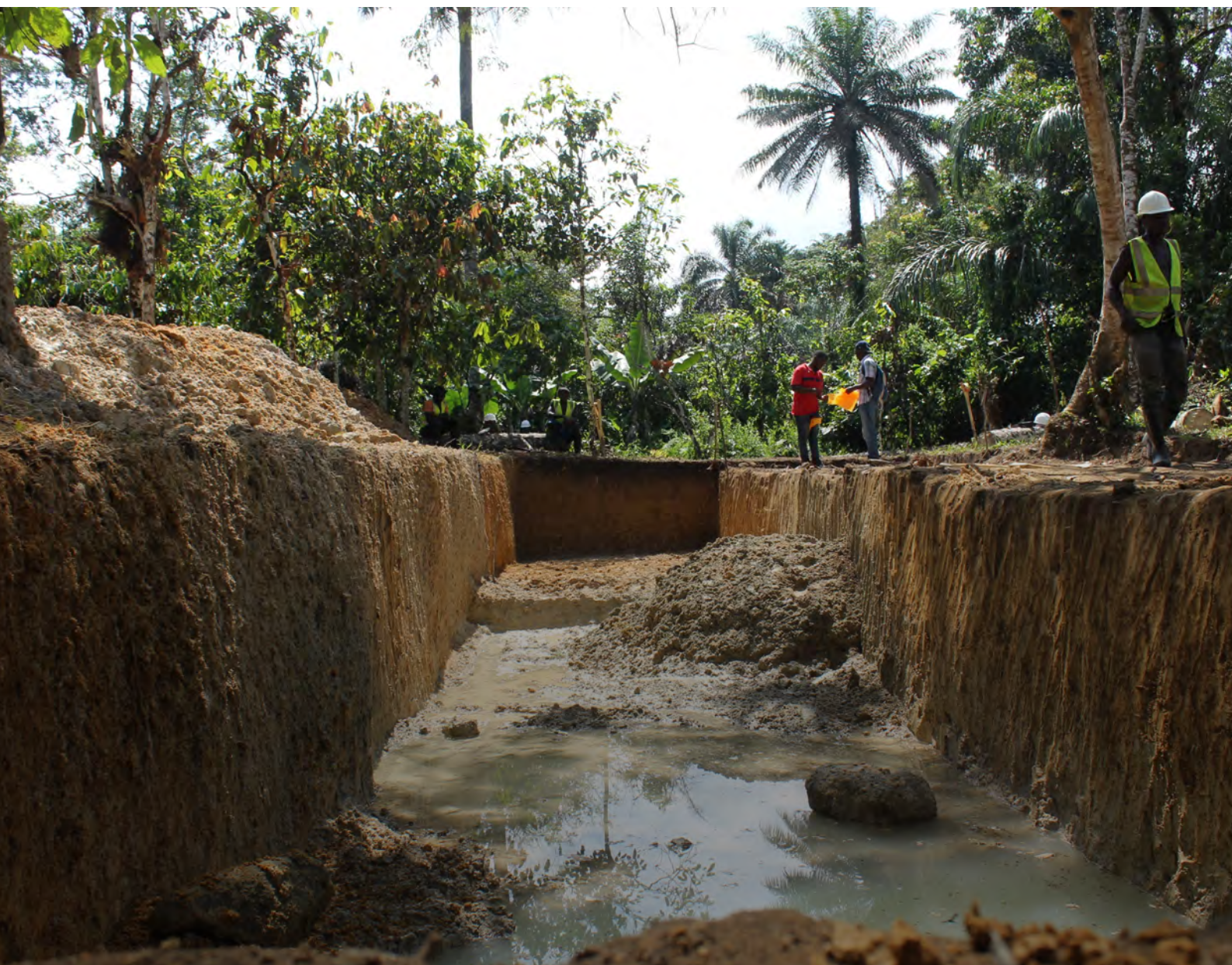
Trenching method in implementation
